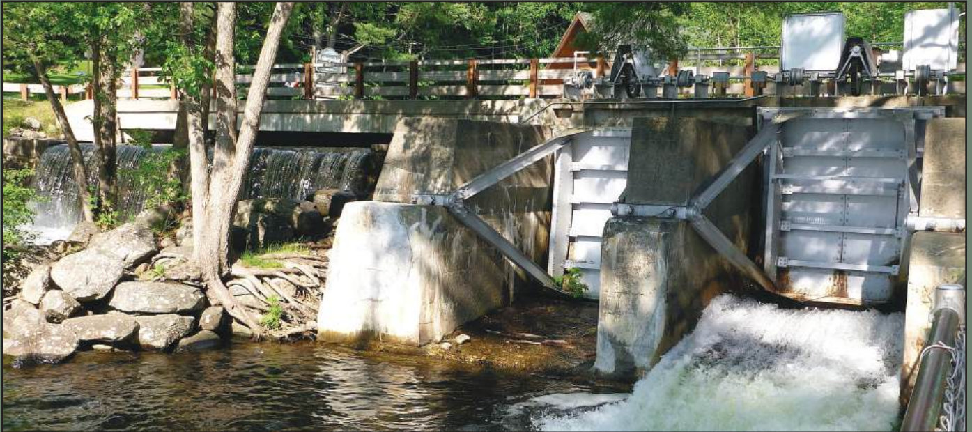
3" flow over the stone spillway
